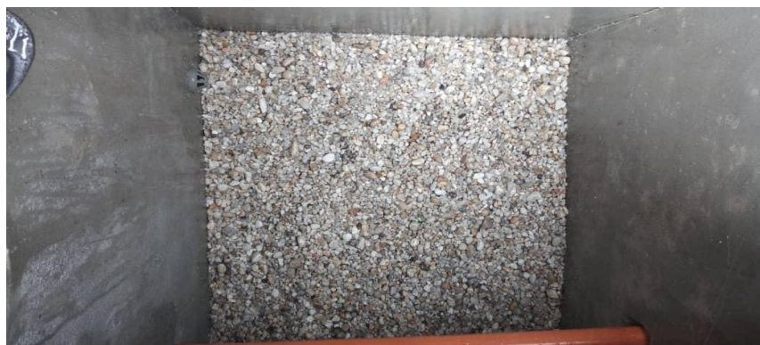
Fig. 10. River gravel (Coarse sand) in the treatment chamber
