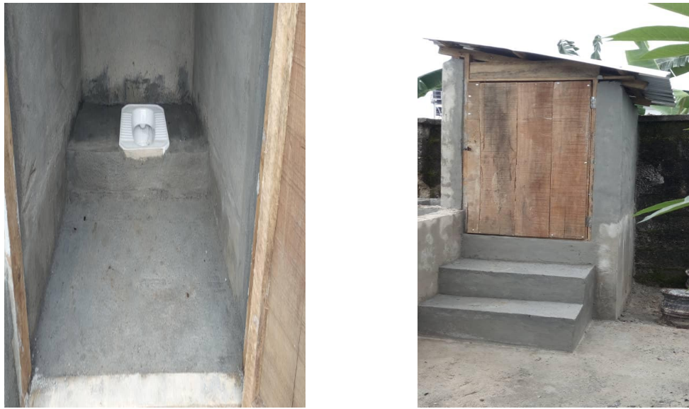
Fig. 4. Inside and outside view of toilet
