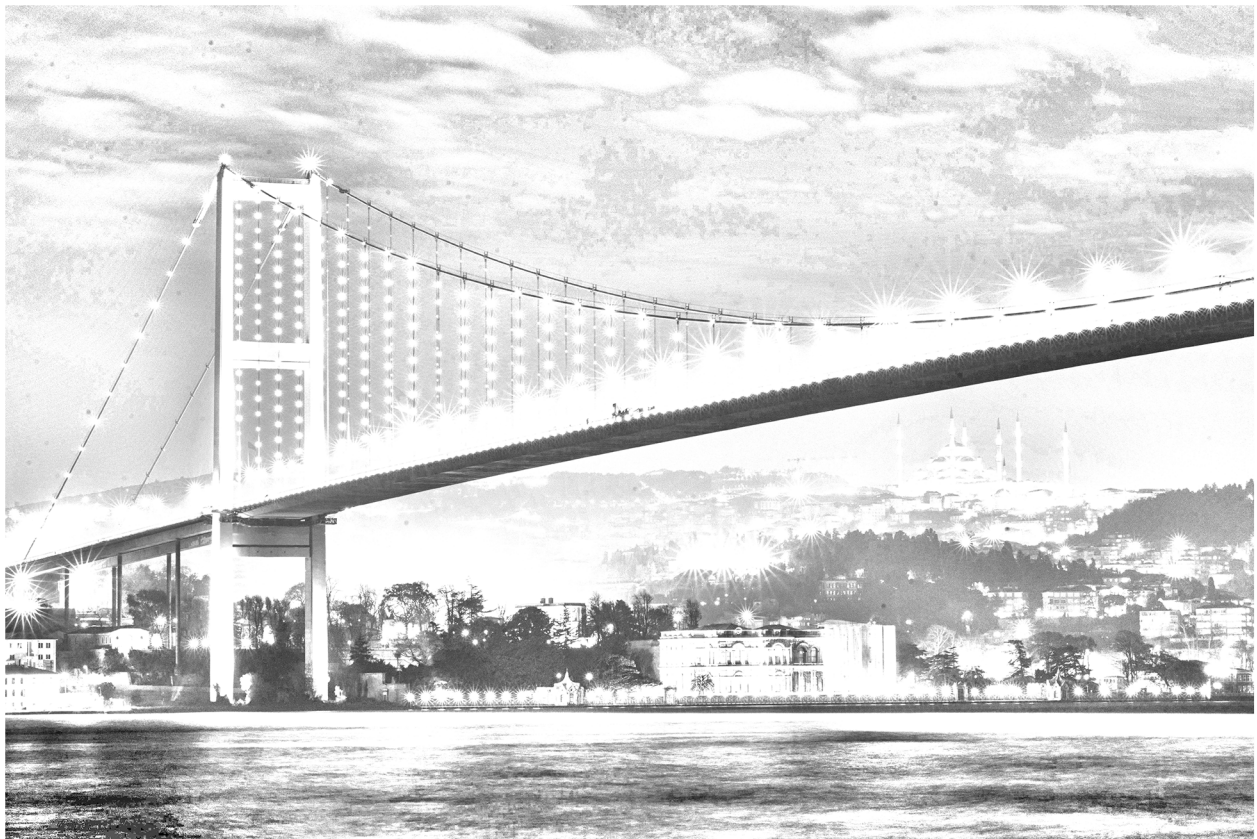
FIGURE 6 Bosphorus bridge in Istanbul, Türkiye shows the idea behind the sling-bridge technique.
