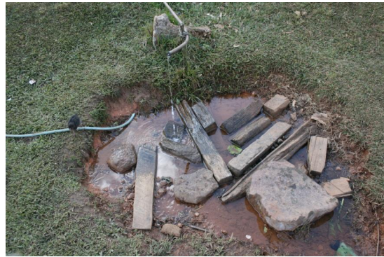
Plate 3. A source of water supply (water pipe) in Nongtynniaw
