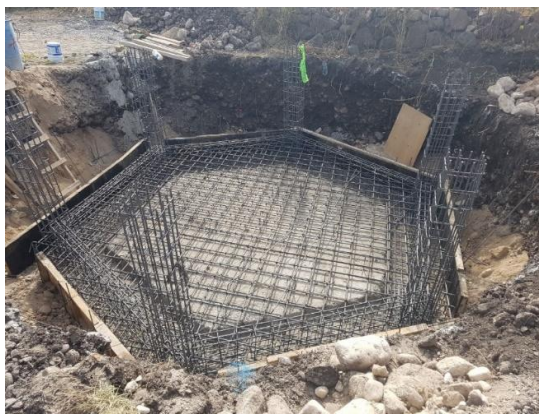
Fig. 3. Concrete Foundation of UAQ's tower
